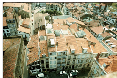
图8 高度密集的巴约纳历史城区 Fig.8 High density of Bayonne historical city center
